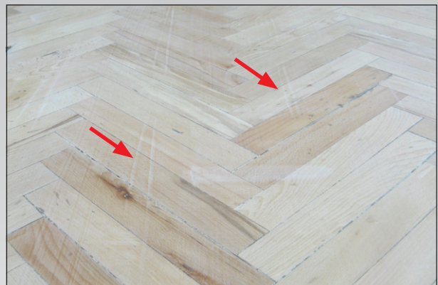
Pic. 4 Grooves in the floor
