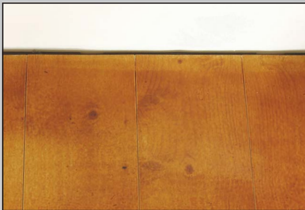
Pic. 17 Old coat (from shellac) on old floorboards.
