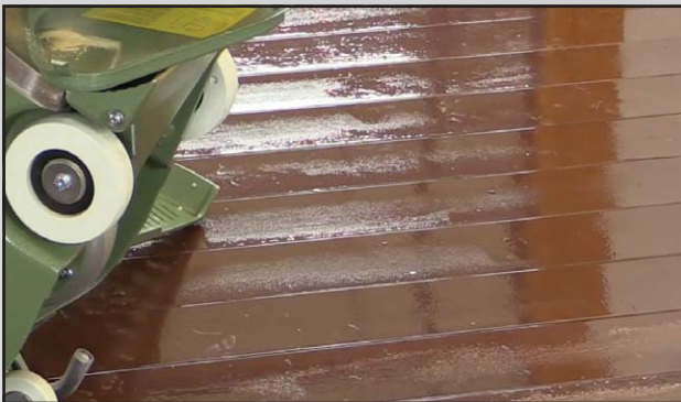
Pic. 3 Easy to see: serious cupping of the floor.
