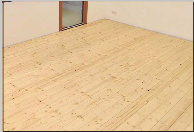
Pic. 18 Finished, oiled surface.
