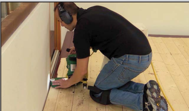
Pic. 11 Sanding the edges with 24 grit.
