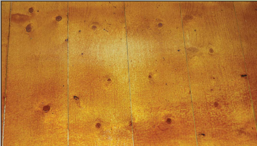
Pic. 1 A thick layer of lacquer on floor boards.
