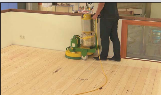
Pic. 12 Removing the milling marks with the TRIO.
