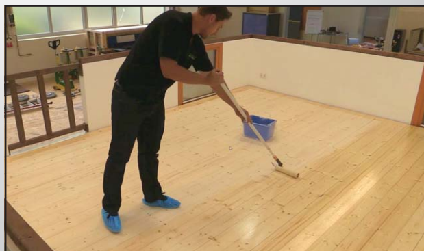
Pic. 15 Rolling on the oil.
