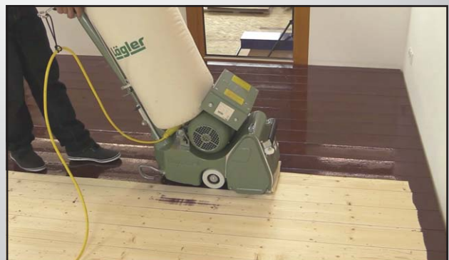
Pic. 7 Milling the surface.
