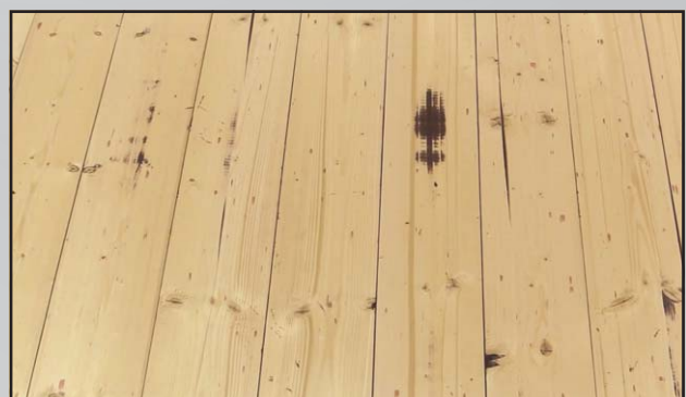
Pic. 8 The vacuumed floor after milling.
