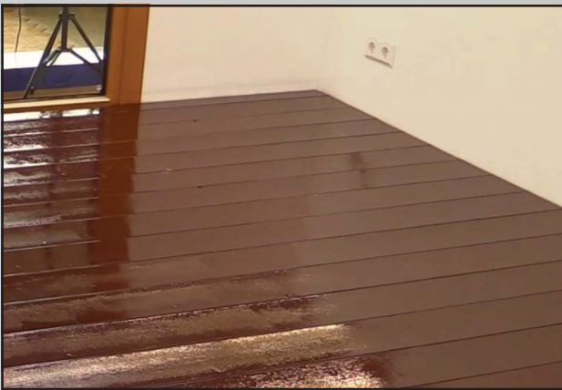
Pic. 17 Cupped, lacquered surface prior to treatment.
