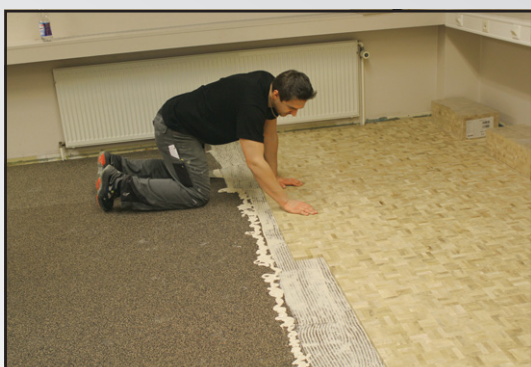
Pic. 10 Laying the new hardwood floor
