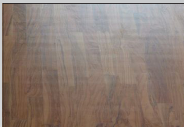
Fig. 3 Waves caused by a NON LÄGLER® sanding drum
