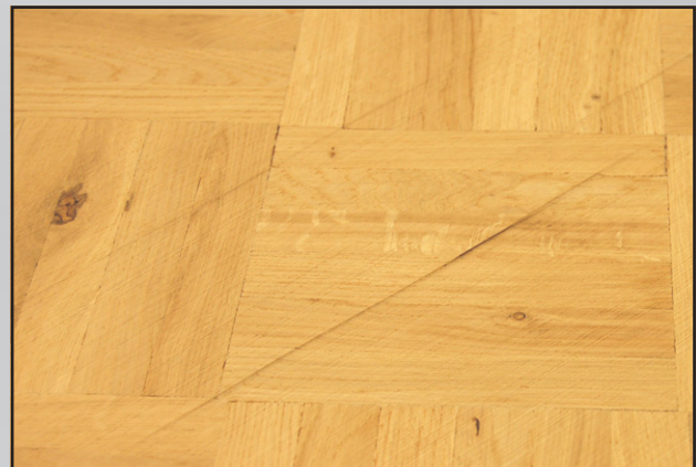
Pic. 7 Side cuts, caused by a flat sanding drum
