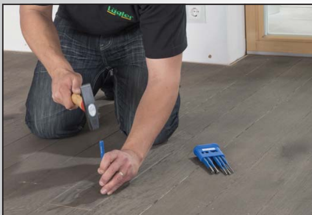
Pic. 7 Countersinking nails
