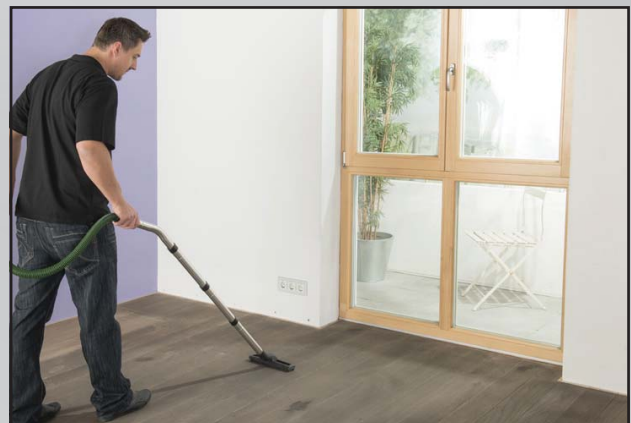
Pic. 8 Very important: always vacuum before each cut
