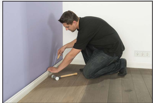
Pic. 6 Removal of the baseboard
